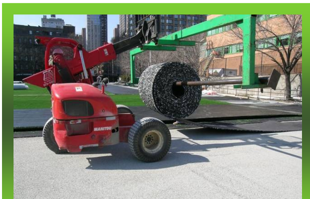
Installation of Sport Shock on Asphalt to Green project, NY 2010
